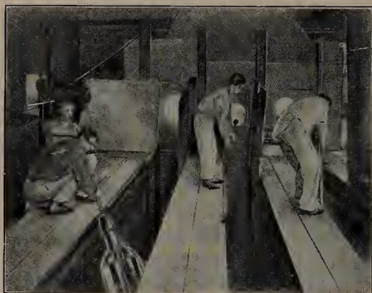
FIG. 151. Second step in making window glass: blowing the cylinders
